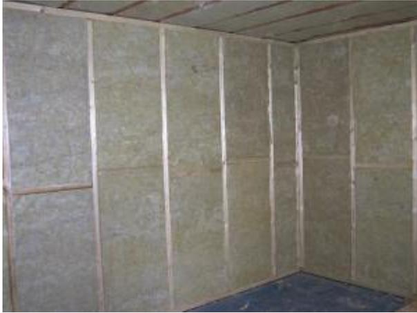
Infill with the supplied [AMW acoustic mineral wool](#) of suitable thickness to fill the void. It does not matter if the AMW touches the wall behind but it must not protrude beyond the surface of the stud. The AMW does not require fixing but should be a loose fit.
