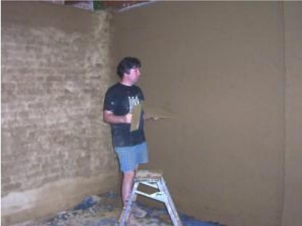
Ensure the wall to be treated is flat and even and remove skirting boards. If it has been 'wet' plastered, tap it to check the plaster has not 'blown' This is when the plaster is coming away from the wall and will sound hollow. It may also 'give' when pressure is put on it. If blown plaster is found it should be chipped off and replaced before any further work commences. Also see notes at the end of these instructions.
