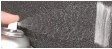
Using our special aerosol contact adhesive (Supplied), bond the [SBM5 sound barrier](#) mat to the plasterboard. The adhesive has an adjustable nozzle so it is usually better to select the widest spray pattern by turning the nozzle so it aligns with the symbol and usually marked H at one o'clock to the nozzle. The other settings are M and L for medium and low spray pattern. (See application instructions on side of can).
