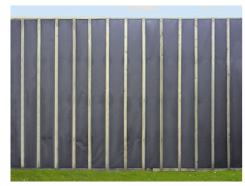
This is the standard or Highway noise barrier but with an extra covering of sound absorption with a weatherproof protective membrane. When applied, the Sound Barrier Extra will improve the acoustic properties of the normal noise barrier fence by an average of 4dB and so can improve an acoustic fence up to 32dB.
