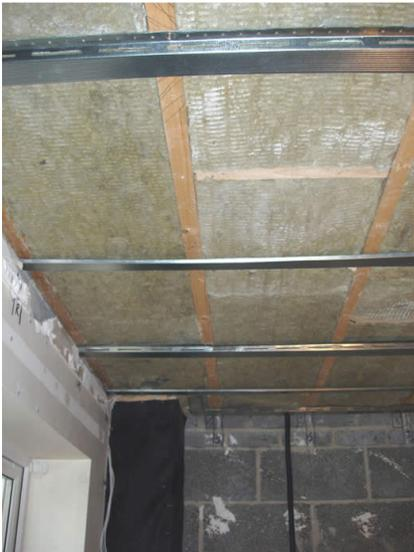
For best results, before the ceiling is replaced, Resilient Bars should be screwed across the joists at 400mm centres as shown above then two layers of high density 12.5mm acoustic plasterboard should be screwed to the bars. An even better result can be obtained if a layer of Acoustic Membrane is sandwiched between the two layers.
