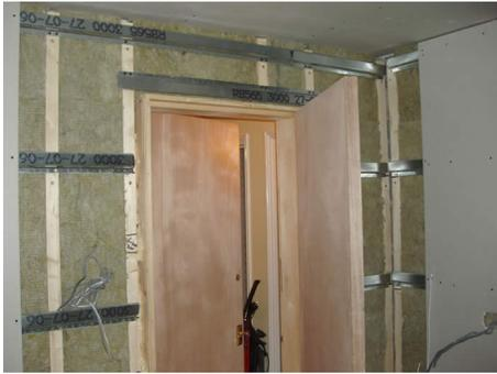
Then install our sound reducing Resilient Bars at 600mm centres across the studwork from floor to ceiling before plaster boarding and as shown in the pic left. To view the technical data on this product please see our Tech Spec page on the website.
