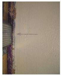
Mark the position of the bars and uprights to help locate them when screwing on the plasterboard. Plasterboard should be screwed to the Resilient Bars with self-drilling screws taking care to avoid hitting the timber stud – **do not screw into the timber stud!**
