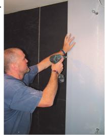
Fix second layer of acoustic plasterboard maintaining the small gap between the floor, walls and ceiling using spacers as necessary. Use the marks previously made to help position the screws and ensure they do not come into contact with the timber frame. Tape and finish off the joints
