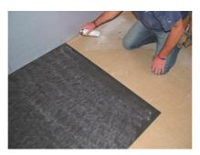
Spray equivalent section of wall for soundproofing mat and also the soundproofing mat with special aerosol adhesive
