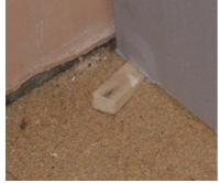
Screw on first layer of acoustic plasterboard with a small gap around the edges of the floor, walls and ceiling using spacers at floor level as shown
