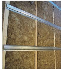
Install Resilient Bars at 600mm centres from floor to ceiling
