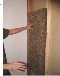
Insert Acoustic Mineral Wool into all of the wall between the timber studs
