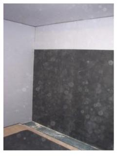
plasterboard. Take care to follow the instructions printed on the sealant cartridge. If this second layer of plasterboard is taper edged then the joints can be filled and finished before decorating otherwise you have to have the boards plaster skimmed first.
