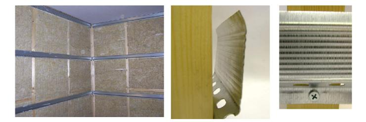
Screw the <u>Resilient Bars</u> (Supplied) across the stud ensuring there is one at the bottom and another along the top then install the remainder between at 600mm centres.
