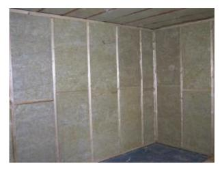
Infill with the supplied <u>AMW acoustic mineral</u> <u>wool</u> of suitable thickness to fill the void. It does not matter if the AMW touches the wall behind but it must not protrude beyond the surface of the stud. The AMW does not require fixing but should be a loose fit.
