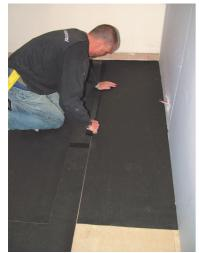
For best results, glue or loose lay SBM5 Soundproofing Mat over the entire floor area to seal up the joints (optional)
