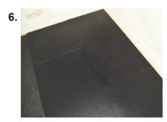
Once the perimeter strips have been fixed, install QuietFloor PLUS panels with the joints tightly butted together
