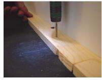
Screw down Perimeter Strips around the edges of the room. The carpet grippers are installed on top of these to allow for the extra thickness of the QuietFloor PLUS
