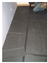
When the floor is entirely covered with soundproofing mat, tape all of the joints using our jointing tape
