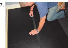
Once the QuietFloor PLUS has been installed, tape up the joints using our jointing tape to ensure the joints remain tightly butted. Now the carpet can be installed directly on top with no additional underlay.
