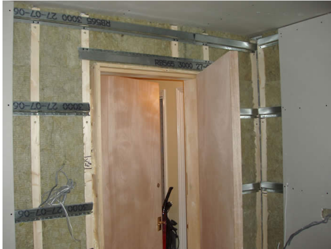
Resilient bar System on a wall before plasterboard layers.
