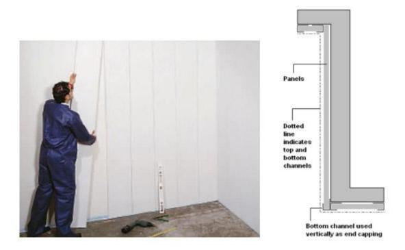
**Walls:** Use a spirit level to align all horizontal and vertical surfaces. Odd leg 'U' channels are plugged and screwed to the wall. Insert the panel into top channel and push panel flush to wall then lower into bottom channel. Use bottom channels vertically as capping to cut wall ends.
