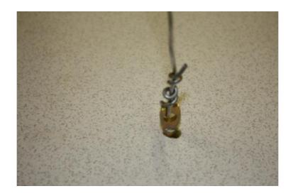
Step 5 – Adjust the height of the cable or chain to suit the depth of suspension required and ensure that the panels are horizontal and level using spirit level.
