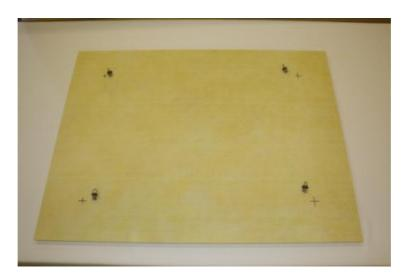
Step 2 – Screw the appropriate number of spiral hooks into the marked positions through the back of the acoustic panel.
