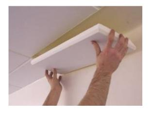
In normal room temperatures, an immediate bond is obtained when sticking the panel so it is important to align the product correctly before pushing the panel into place. It is important the adhesive has reached the correct stage of tackiness before applying a tile.
